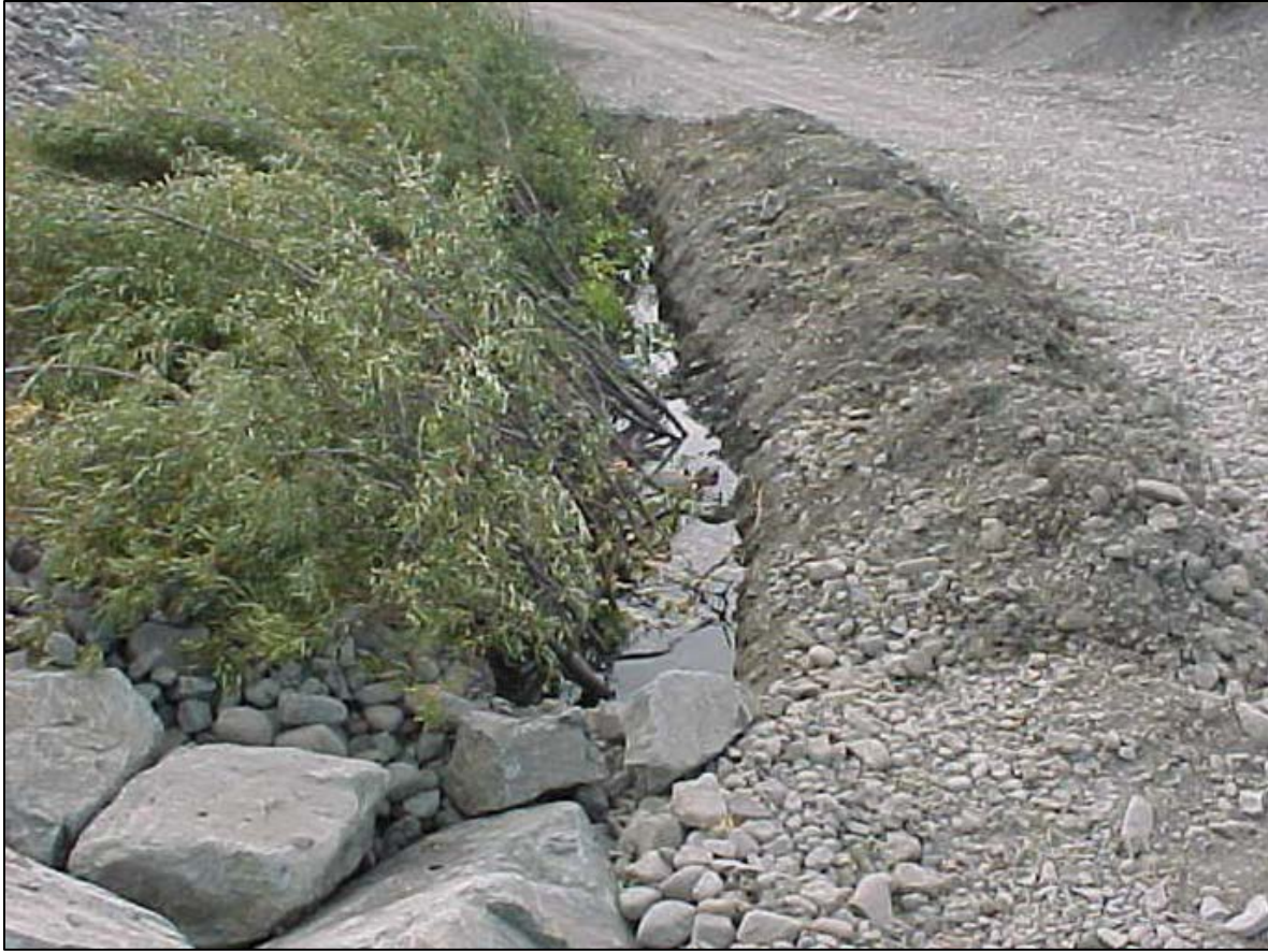
Figure 5. Willow wall planted in wetted trench adjacent to where surface flow goes subterranean.
