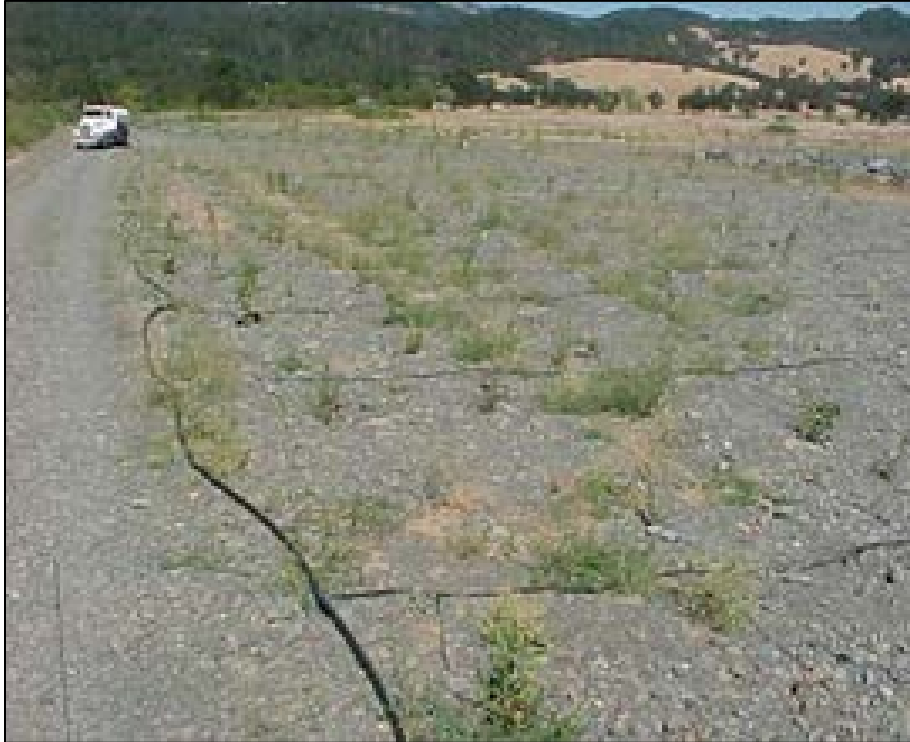
Figure 6. Waterline System for Watering Large Areas
